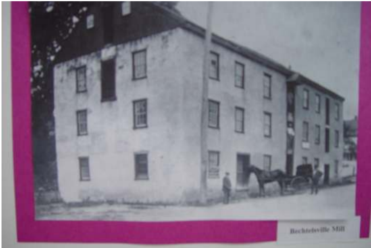
This stone/stucco mill of 3.5 stories, the top 1.5 stories being of wood frame construction, was built in 1820 and operated for a time as a linseed oil mill known as Bechtel's Oil Mill.
